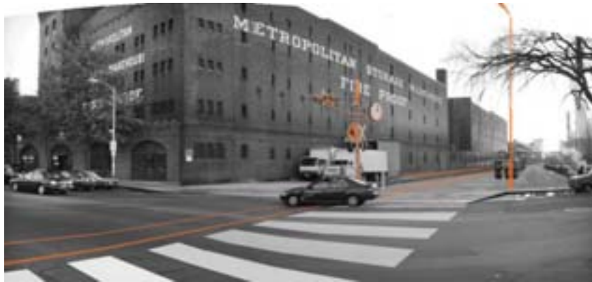
Massachusetts Avenue crossing
