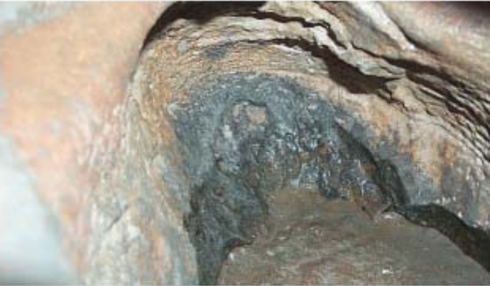
Close-Up View of Cavity
