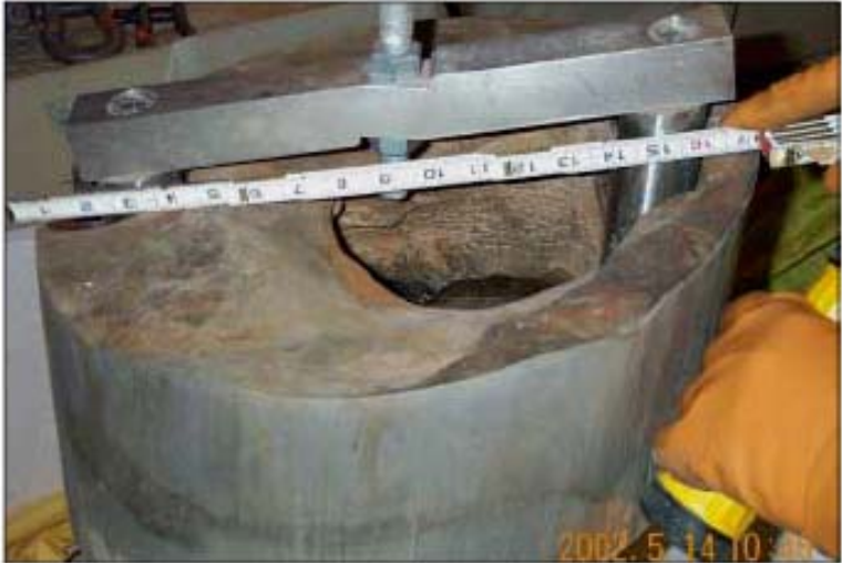
Nozzle #3 Area Cut Away From Reactor Head
