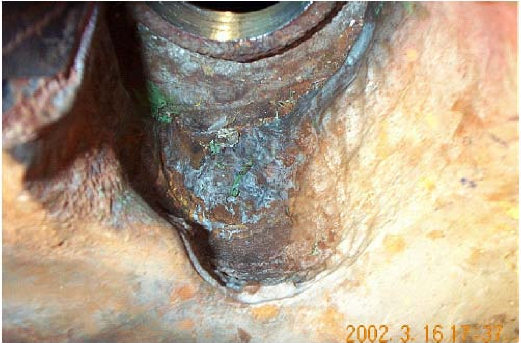
Nozzle 3 with insulation removed and shielding installed 03-16-02
