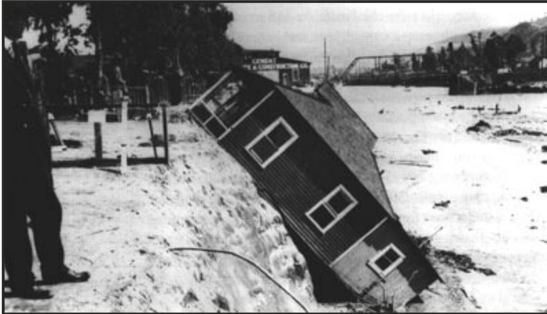
A house collapses into the riverbed following the 1914 floods. (Gumprecht)
