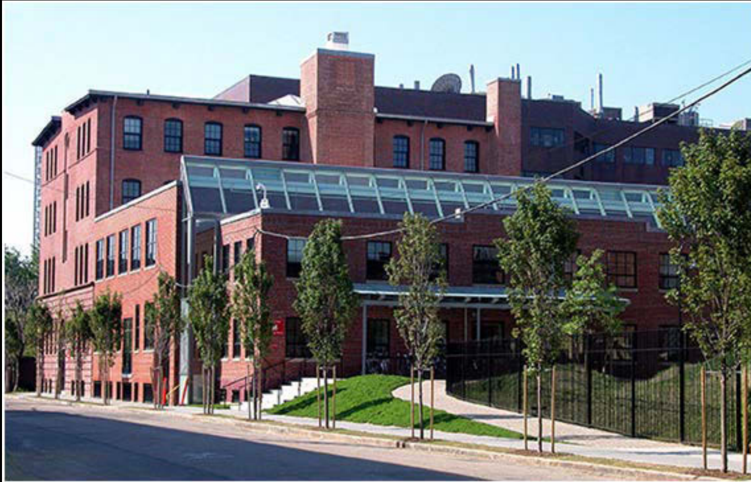
Blackstone Building (architecture: Bruner Cott)
