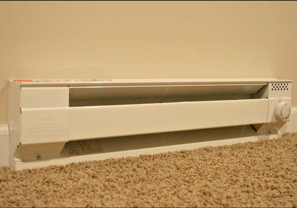
Electric baseboard heater
